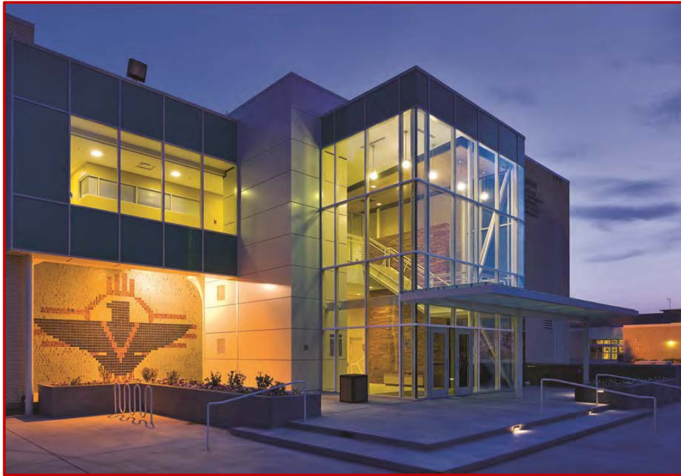
New Mexico Junior College Pannell Library Addition and Renovation Photo by Patrick Coulie Photography
